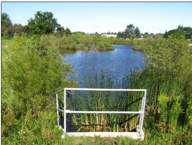
Figure 9-3: Turnberry Drive SWMF outfall.
