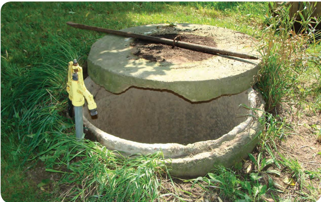
FIGURE 1: DAMAGED LID AND CASING
