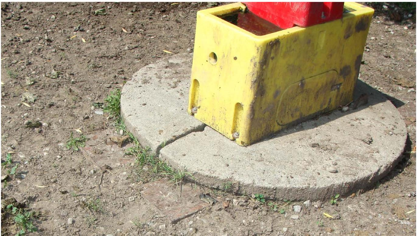
*This picture shows the gap in the concrete well cap and its location in relation to the ground and potential sources of contamination.*
