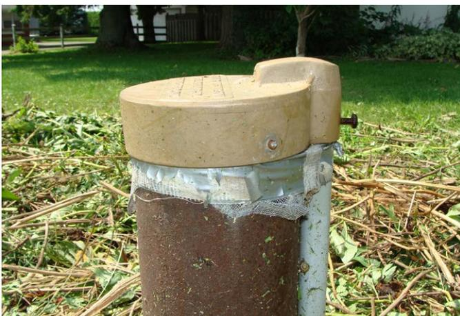
*An inadequate well cap may allow pests and other types of contamination to enter into the well, and may not allow for proper ventilation.*
