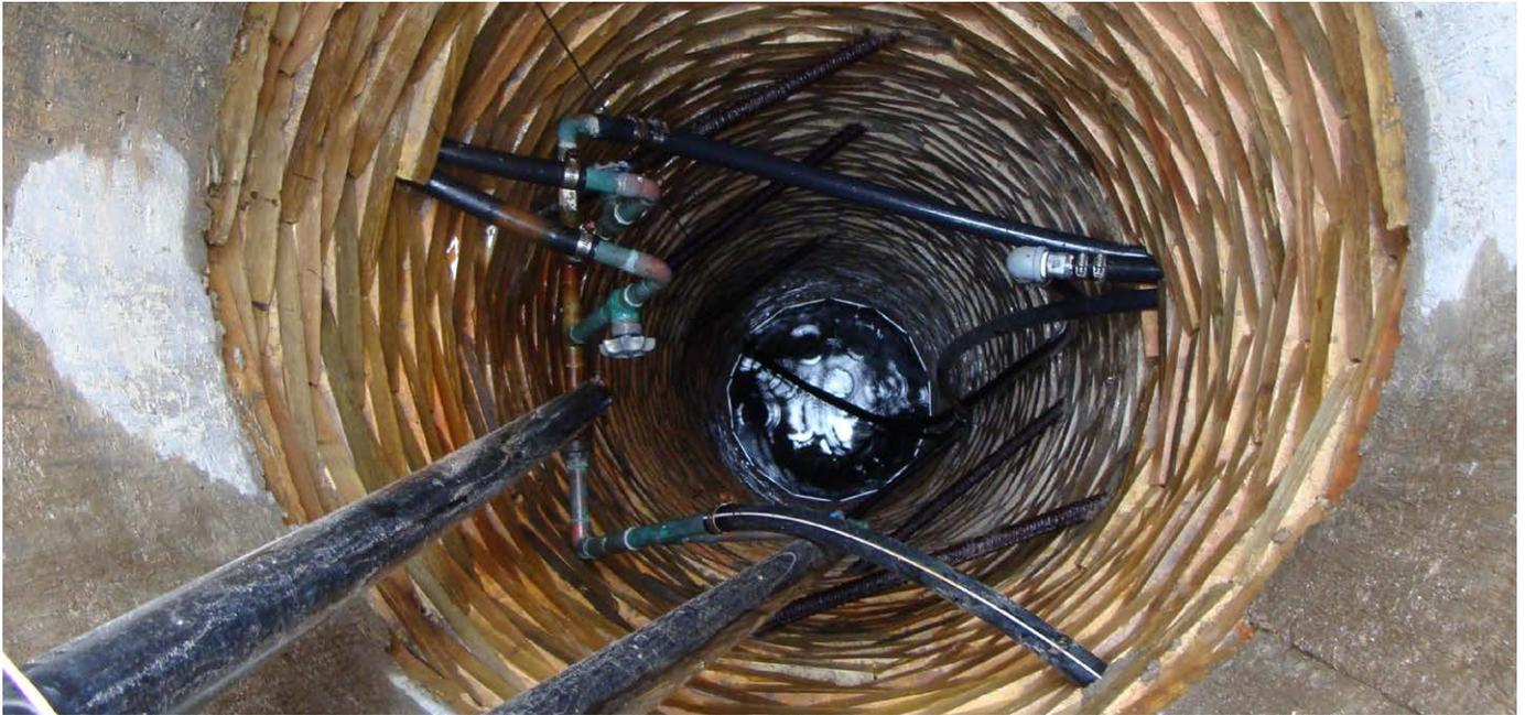
*A dug well that is over 100 years old. Moisture seen on the concrete and tile casings indicates that surface water is getting into the well. Ensure that the well is constructed and maintained properly to reduce potential contamination from entering the well.*
