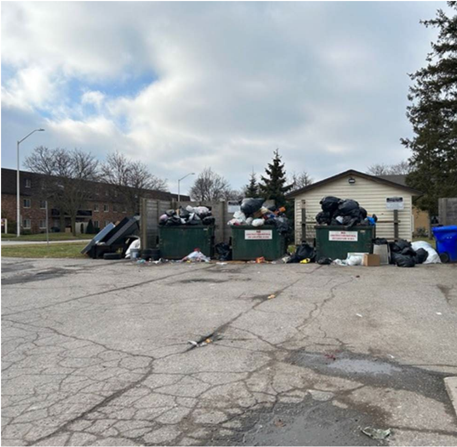
Property Maintenance Violation
